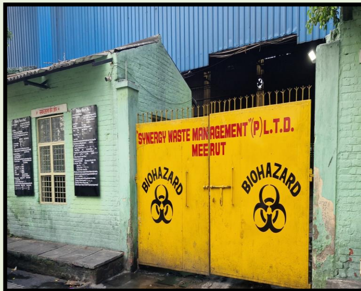
Biomedical Waste Treatment Unit
